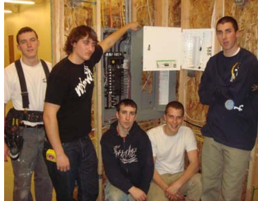
Residential graduates finishing up their craft certification dog house. Pavel Lutsyuk, Max Ladenburg, Jordan Shumate, Spencer O’Galleher and Mark McGunagle.
